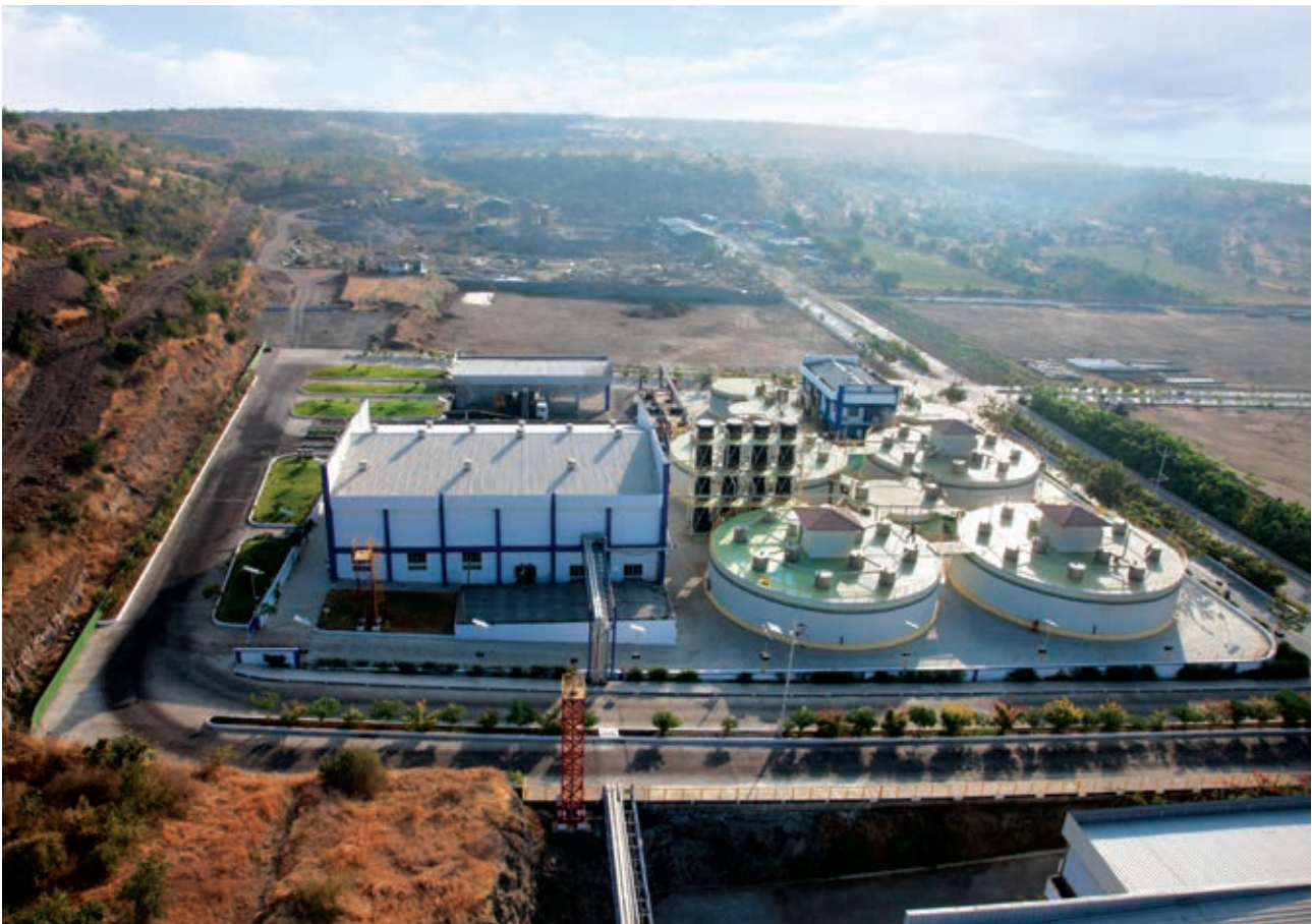
1.6 MW Bio-gas power plant
